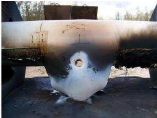
IMPACT NOT COMPLIANT
