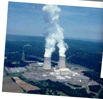
The Susquehanna Steam Electric Station , a boiling water reactor
