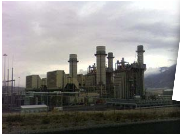
Currant Creek Power Plant near Mona, Utah is a natural gas fired combined cycle electrical plant.
