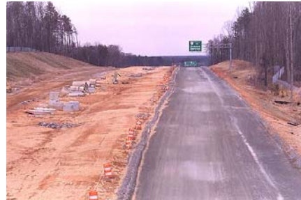
Poor lane markings
