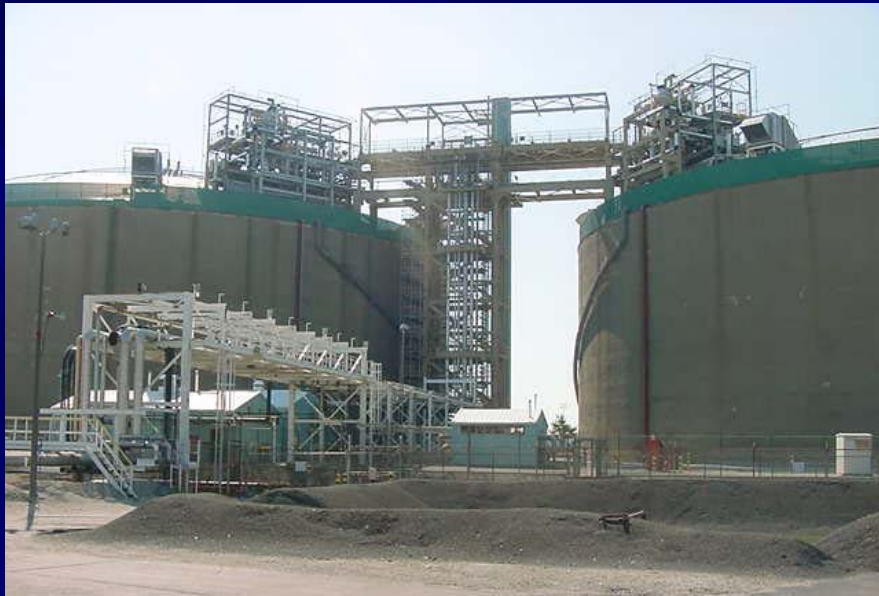
PGW PORT RICHMOND PLANT
