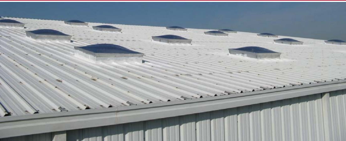
JSC Gilruth Center Daylight Harvesting Fixtures
