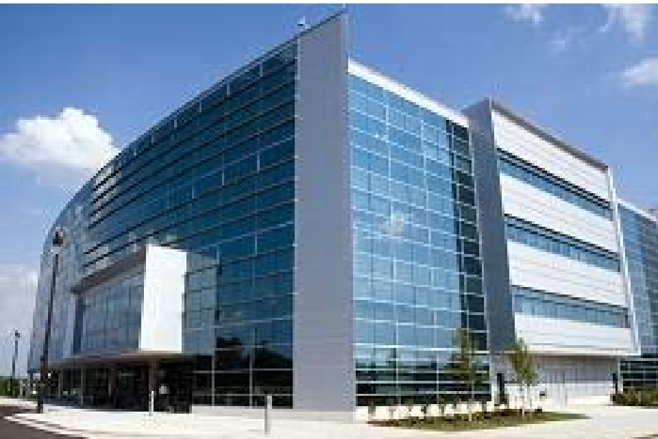
MSFC Building 4601, Office Building - Gold
