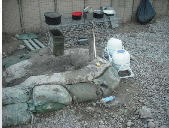
Well Installed On FOB by Local Afghans
