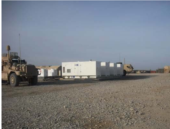
Dependent on Contractors (Major FOBs completely dependent)
