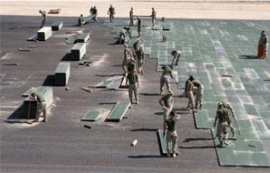
Marines attached to the 24th Marine Expeditionary Unit, lay down AM2 matting while in Kandahar Province, Afghanistan.
