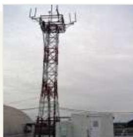
A 1-kW fuel cell system has been providing power for this FAA radio tower near Chicago for more than three years.
