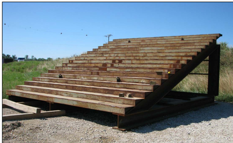
Construction of Staircase
