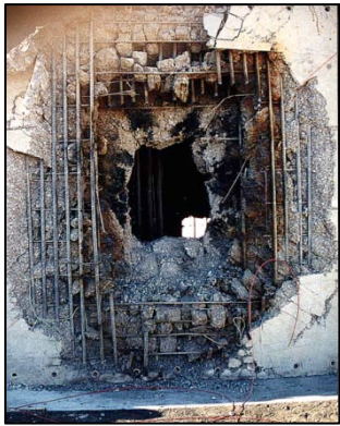
Concrete breaching
