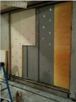
Testing Hi TL Bulkhead
