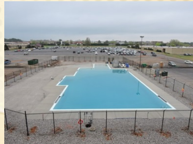
SWCS Test Certification Center
