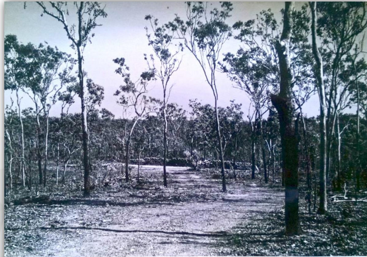
8. FIRST BLOW (SEE PICTURE No.9)
