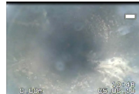
Inside of the explosive hazard pipe after treatment
