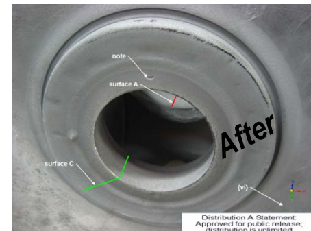
TD-63 Actuator repair
