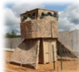
Multi-Purpose Guard Tower
