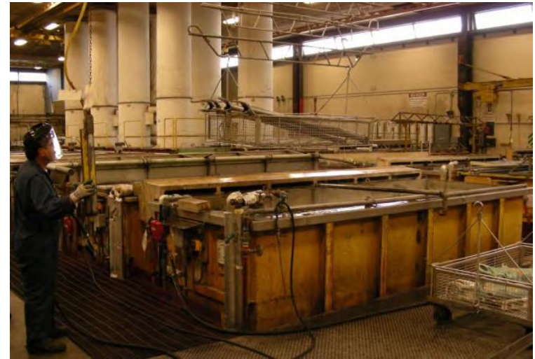
Immersion Paint Stripping Tank (Photo: M. Huber, DoDREC9 PM, brief to Cal EPA & DTSC, 27 Oct 2014.)
