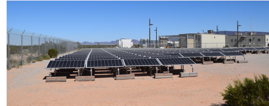
Border Patrol FOB - Split Phase Site Load - Avg 25 kW with 45 kW peak
