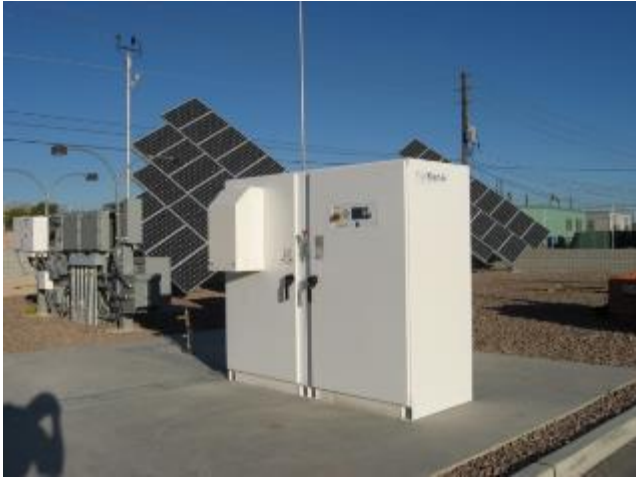
Proton electrolyzer producing hydrogen from solar power
