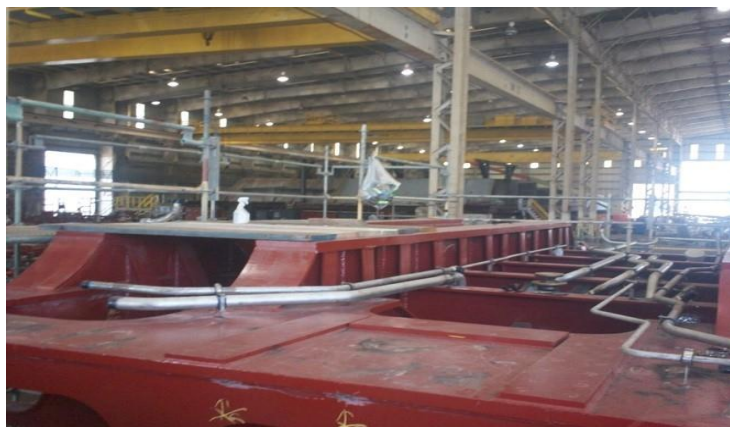
Main Propulsion Diesel Engine Foundations
