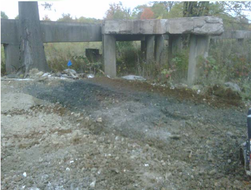
Left: MuniRem Mixed in with Soil but No Water Added Yet.
