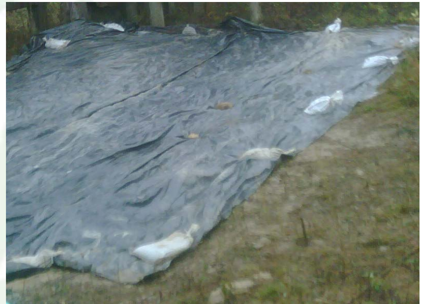
Right: MuniRem Mixed in with Soil, Water Added and Covered.
