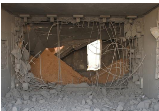
a. Internal view of test wall 1
