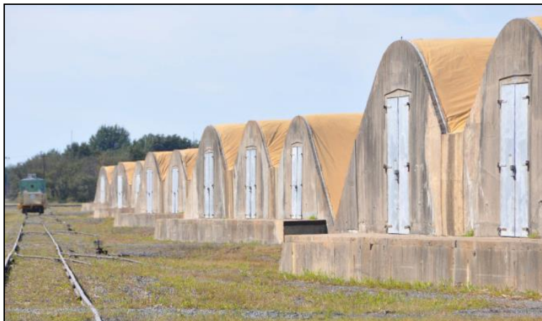
Figure 1 Earth Covered Magazines Pictures
