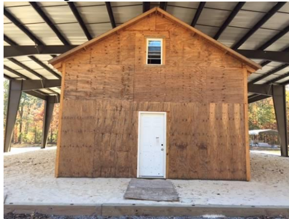
Figure 2-1 – ATF Blast House
