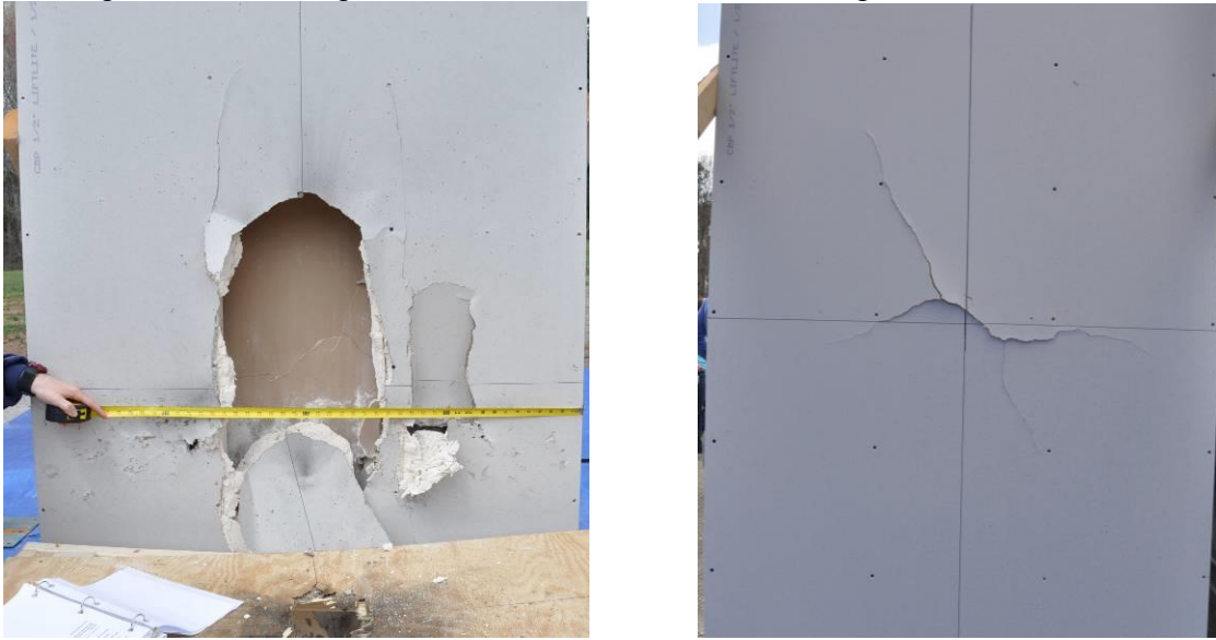
Figure 3-2 – Damage from SQRL Phase II Test 1-2 (40 g C-4, 12” Stand-off)
