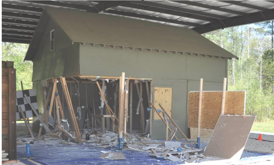
Figure 3-5 – SQRL Phase II, Test 4-1 (250 g, 48” Stand-off, Blast House), Damage to
