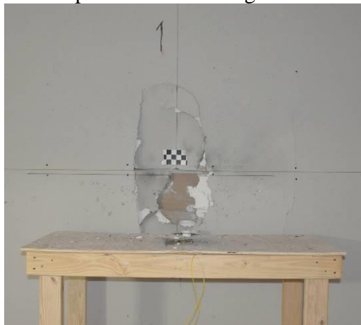
Figure 3-4 – SQRL Phase II, Test 3-2 (30 g C-4, 12” Stand-off, Blast House) Damage to Explosive Side of Target Wall
