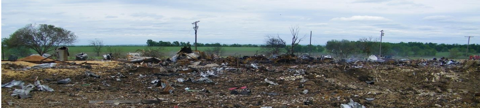
Office / Chemical Storage Building at 85 ft. – K3
