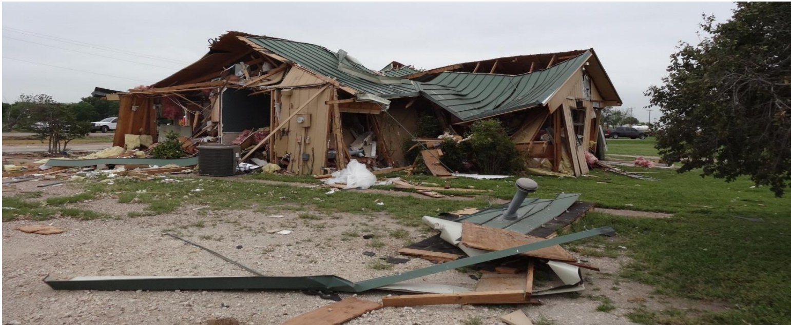
Scale House at 445 ft. – K15
