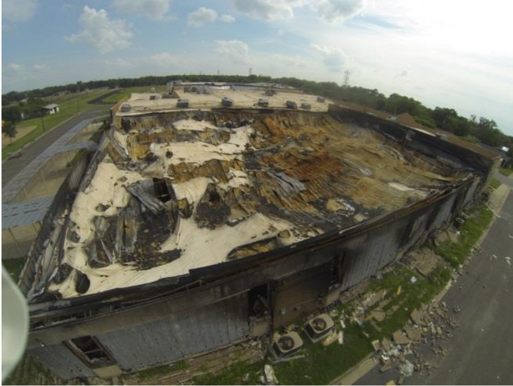
Figure 9. West Intermediate School – Original School Northeast Wing Roof
