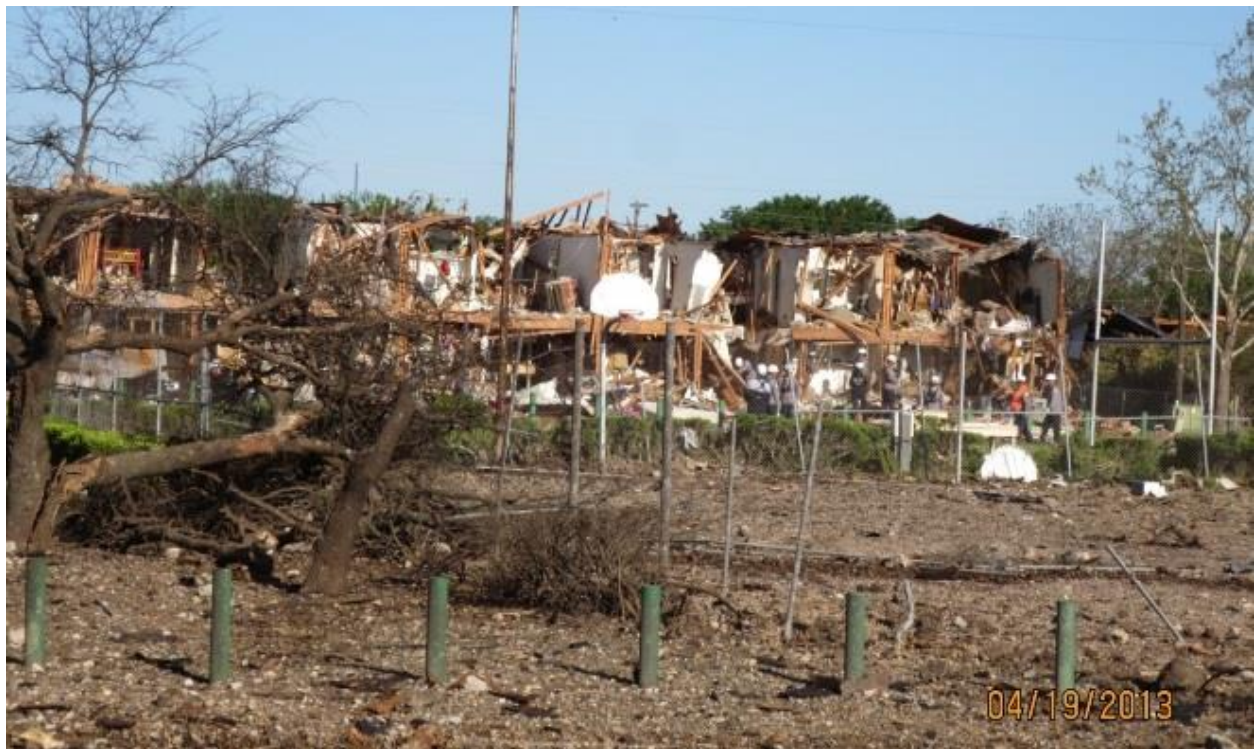
Figure 5. Apartment Complex East Façade – 450 ft. (K15)
