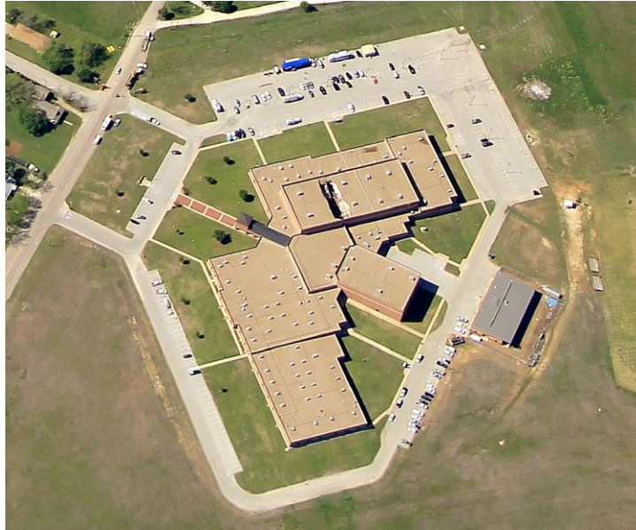
Figure 12. Aerial View of West High School Roof– 1,500 ft. (K50)
