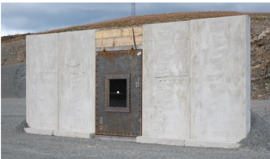
Figure 2 Test structure with chamber and concrete walls 16
