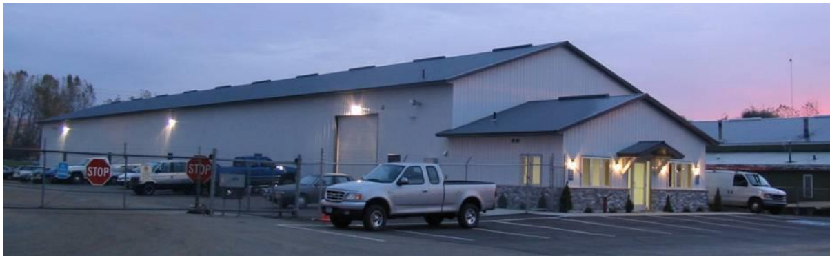
Det-Tronics Engineering Test Center
