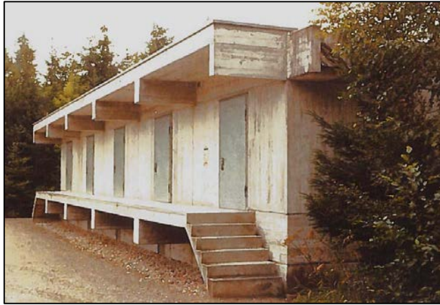
Figure 2: Typical Swiss Above Ground Magazine for Training Ammunition
