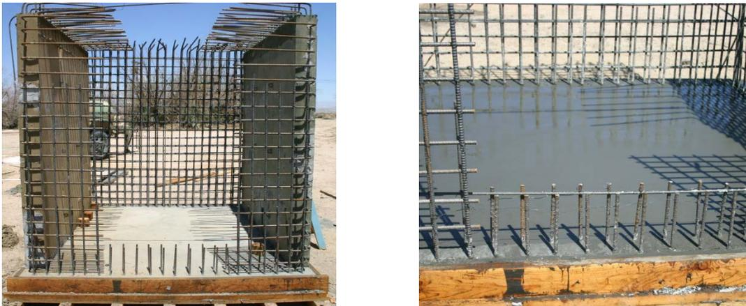
**Figure 1: Construction of Kasun Structure**
