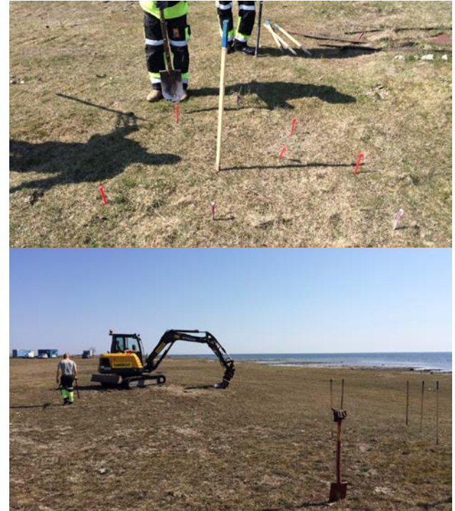
Verification of UXO indications (Södra Sandby, 2016)
