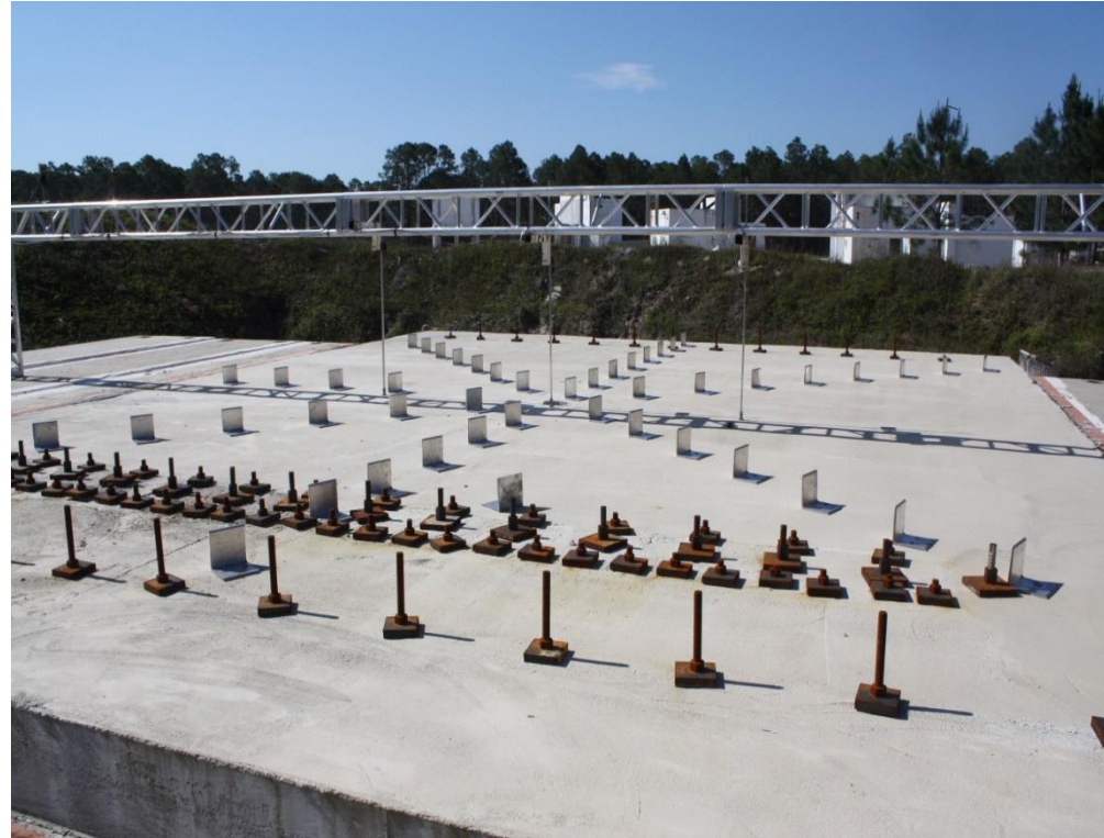
Roof Displacement Gauges
