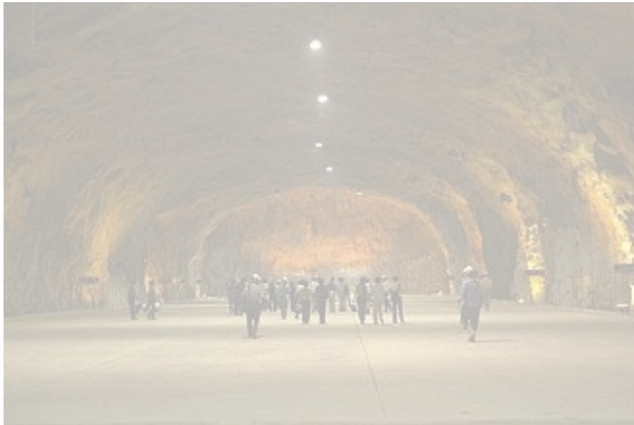
Underground Ammunition Facility
