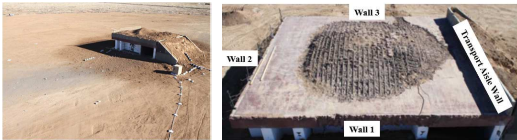
Figure 8 Post-test views of the test structure showing Wall 1 and the roof with (a) soil cover and (b) soil cover removed after the test [7]
