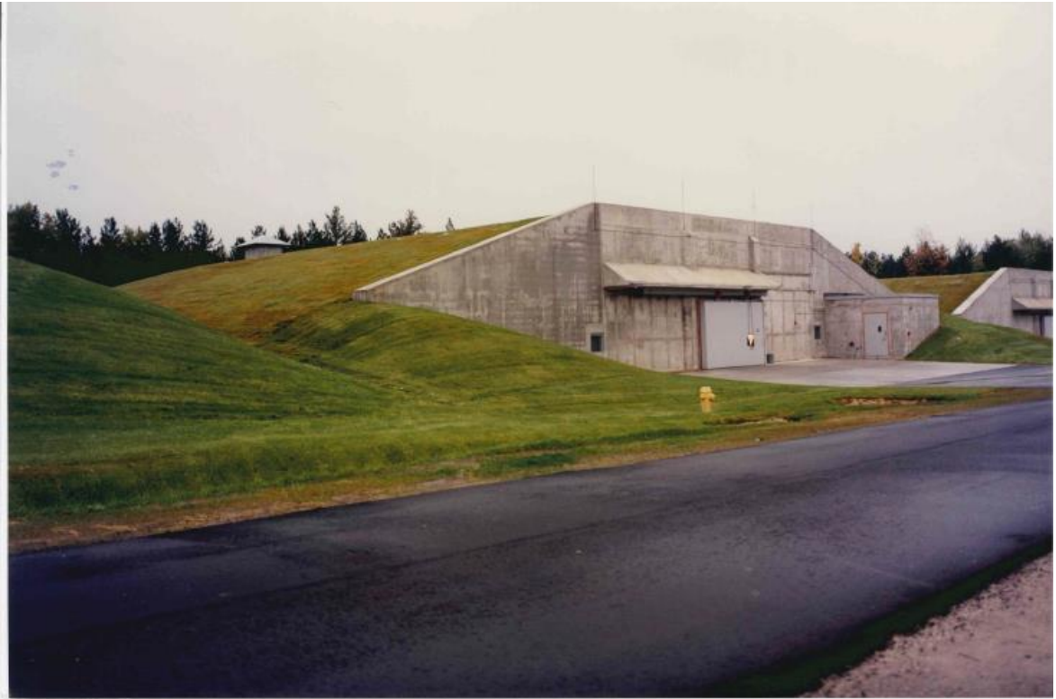
Fig. 1c - CLSECM in summer environment with Annex Structure in the front
