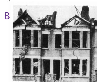
Limiting 'B' damage, with gaping cracks in external walls
