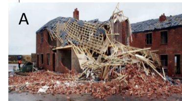
Limiting 'B' damage, with gaping cracks in external walls
