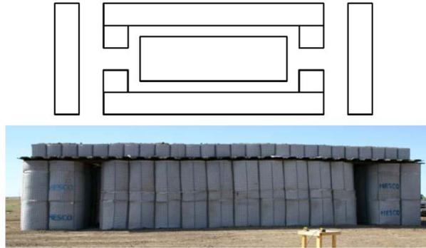
Figure 12. Hardened structure with a flow-through design [Anderson, et al., 2008]
