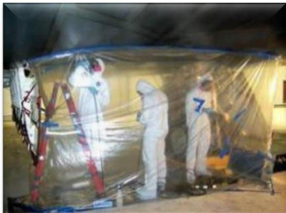
Airmen sanding degraded paint coatings within an enclosure to contain hazardous material generated during de-painting.
