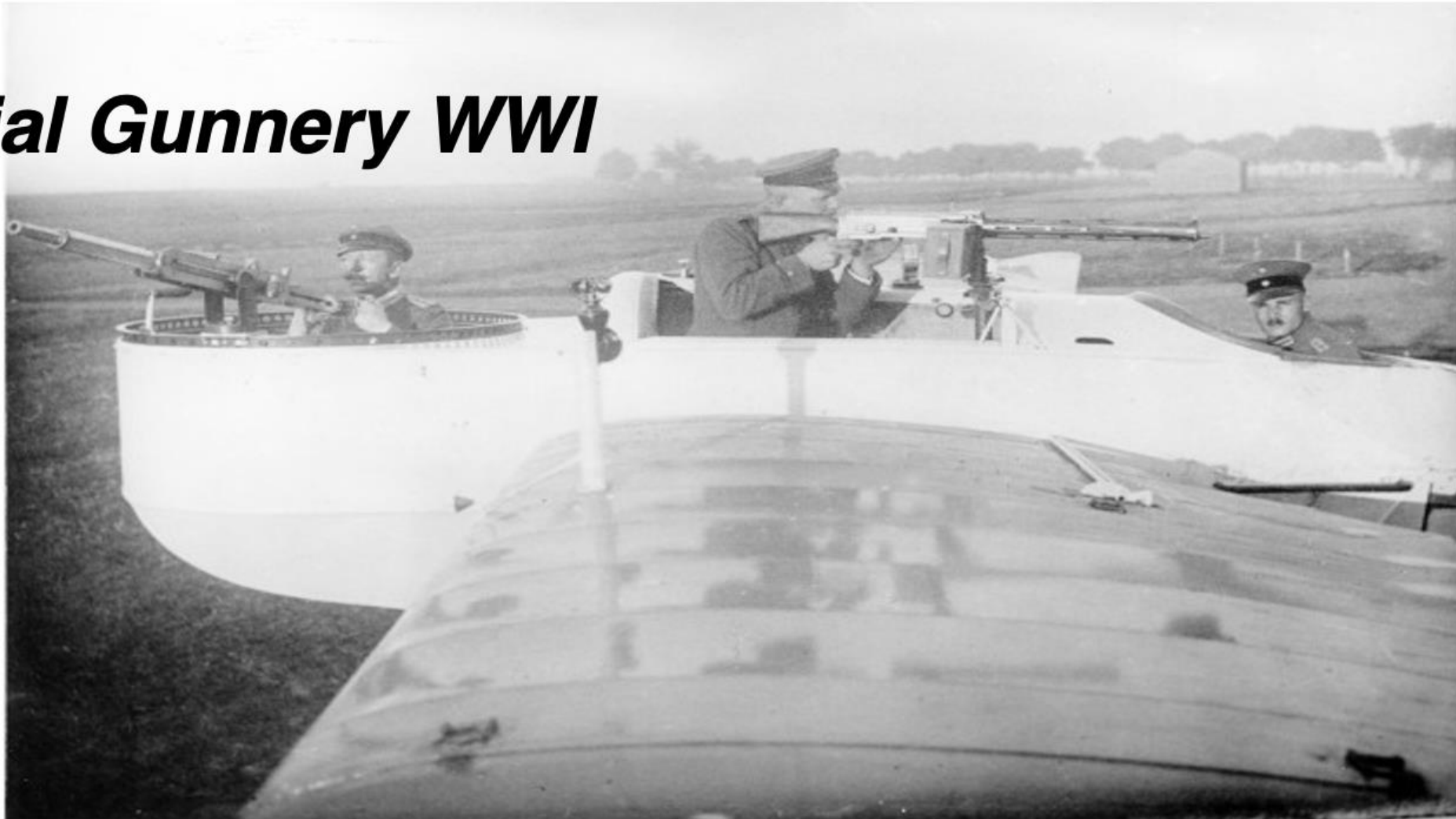
20mm Becker Autocannon in the Front of a Gotha G.1
