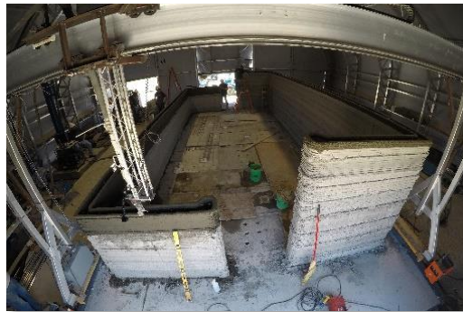
Automated Construction, 3-D printed buildings
