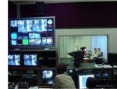
MPC-H Control Room
