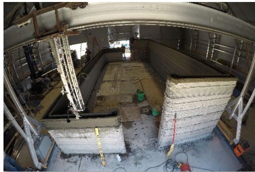
Automated Construction, 3-D printed buildings
