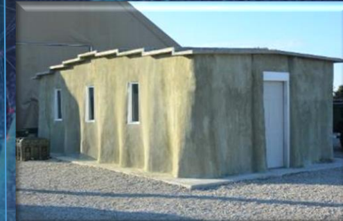
3D Printing of Concrete Buildings
