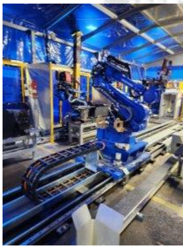
Band Weld Cell Installation at IMT
